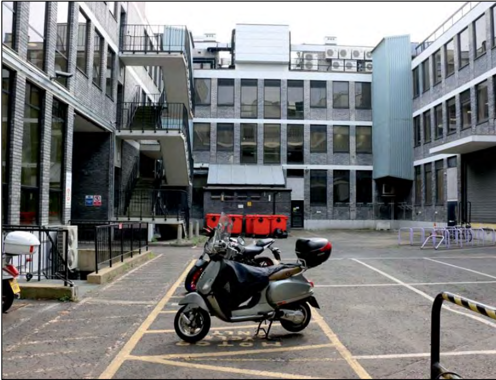
Figure 10: Existing central courtyard
