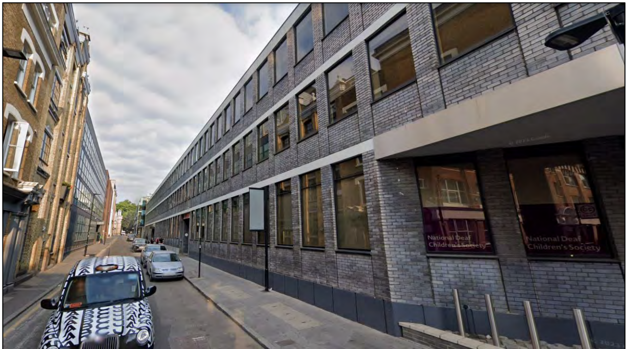
Figure 7: Epworth Street elevation, looking west
