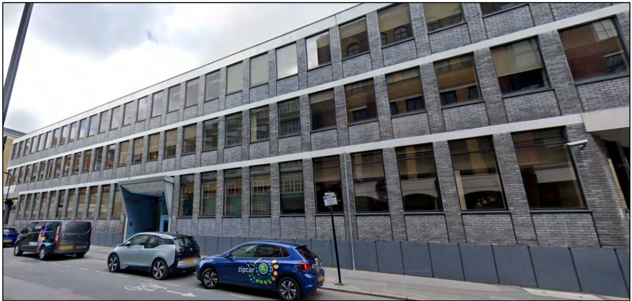
Figure 6: Paul Street elevation, looking south
